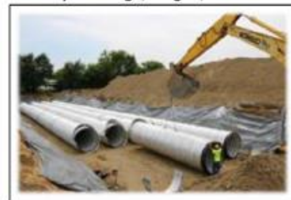
NG Pipe Storage, Erdgas, Switzerland 12
